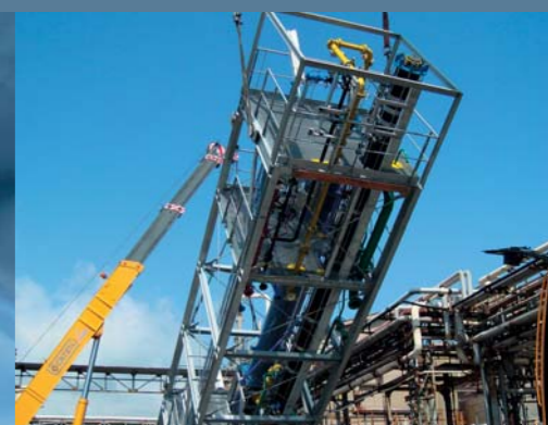
Schlüsselfertige SINTACLOR® Anlage
